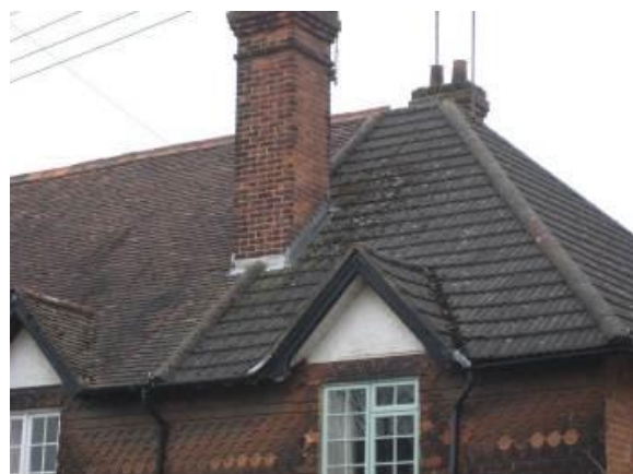
Replacement windows and concrete roof tiles
