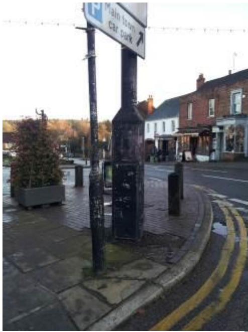
Street furniture in need of maintenance
